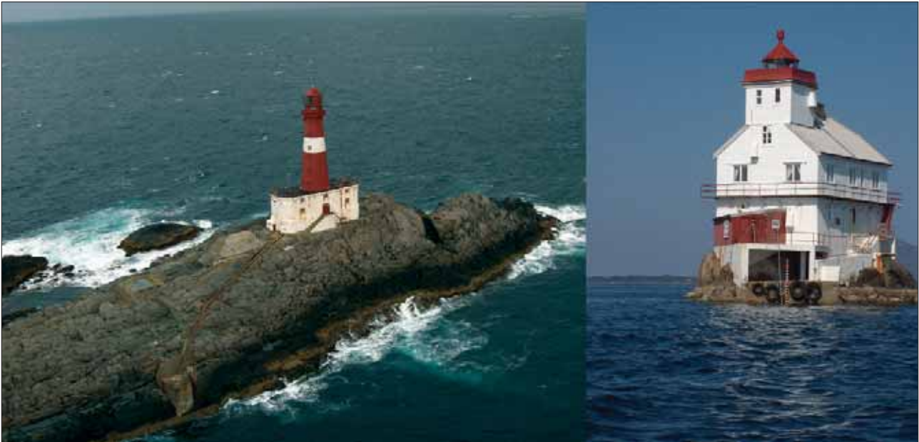
2. - Two of several remote lighthouse stations with hardly any soil. Måløy/Skarholmen station (No) to the left and Stabben (SF).
